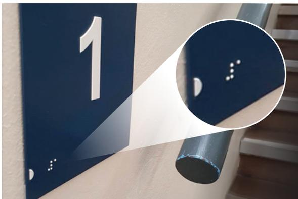
Following concerns raised by a blind member of staff, Braille numbers were applied to the walls, at the end of the handrails where the flight meets each floor level landing in the Tower Block stairwell.
